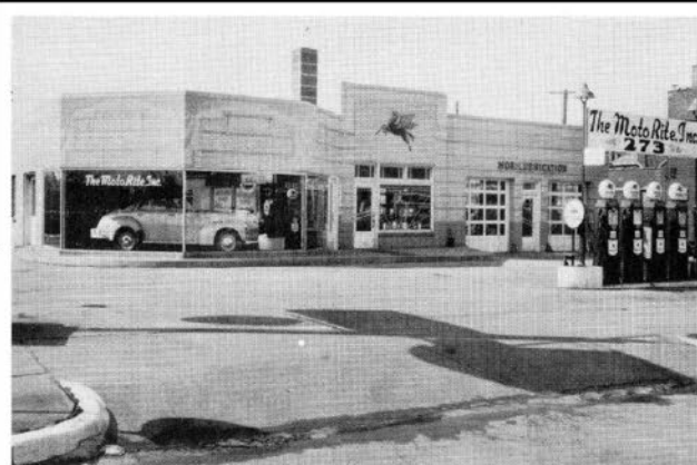
The new location of MotoRite, Inc., Studebaker dealers in St. Louis, Mo., permits a diversification of business that is conducive to consistent profits. Revenue from their modern gasoline station supplements the income from their equally modern service station which includes an excellent parts department, a customer waiting room, two lubrication boists, and four stalls for customer work. A large parking area is provided in the rear. The shadow of the Authorized Service Sign, which is mounted on a post at the curb, can be seen on the pavement foreground. (Parts & Accessory News April 15, 1942)
